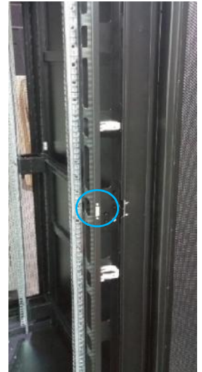
Improved cable management kit with magnetized cover for 26" racks
