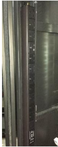
Flushed mounted PDUs!
