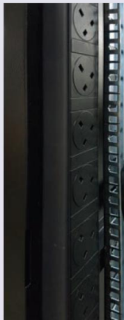
Semi-flushed mounted power distribution units prevents obstruction during rear mounting of equipment
